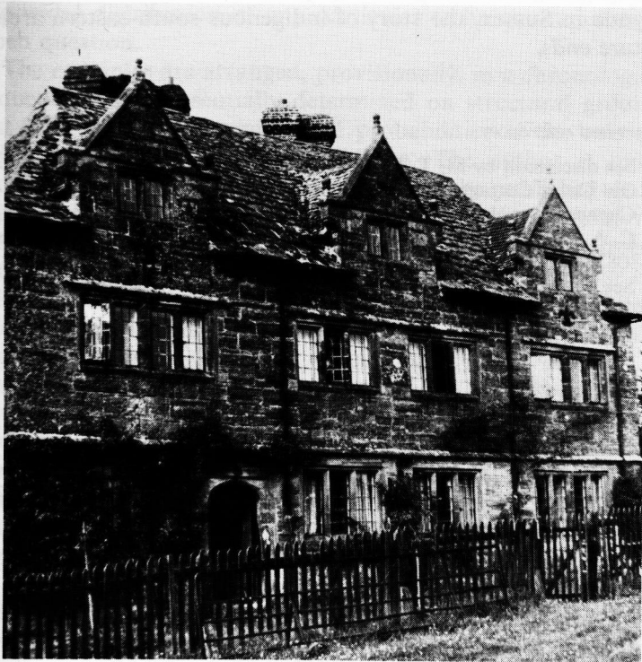
Fig. 10. Gullege. E. Grinstead. Post-medieval Standardisation. The Cotswold-type façade covers a sixteenth-century jettied house
