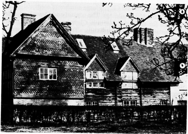
Fig. 8. Camouflage. Fifteenth century hall with Jacobean wing, all concealed by later claddings. Spicer's, Balcombe, Sussex
